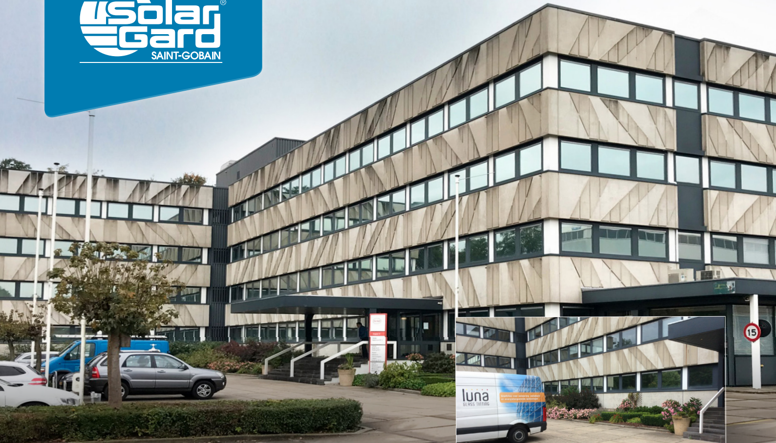
Silver 20 was installed to cut heat and glare
