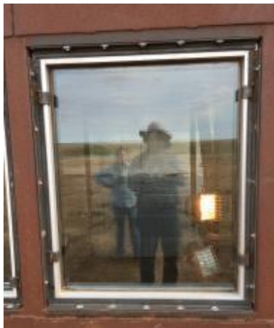
Figure C.5: Specimen 1-2 Pre-Blast Condition Exterior
