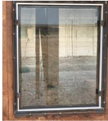
Figure C.32: Specimen 3-3 Pre-Blast Condition Exterior
