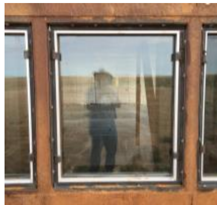
Figure C.24: Specimen 2-3 Pre-Blast Condition Exterior
