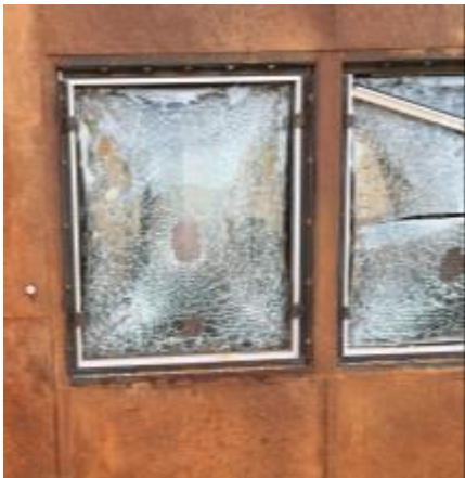
Figure C.21: Specimen 2-2 Post-Blast Condition
