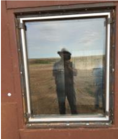
Figure C.1: Specimen 1-1 Pre-Blast Condition Exterior
