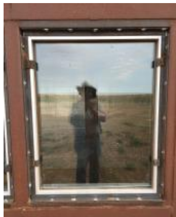
Figure C.14: Specimen 2-1 Pre-Blast Condition Exterior
