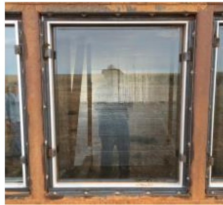
Figure C.28: Specimen 3-1 Pre-Blast Condition Exterior
