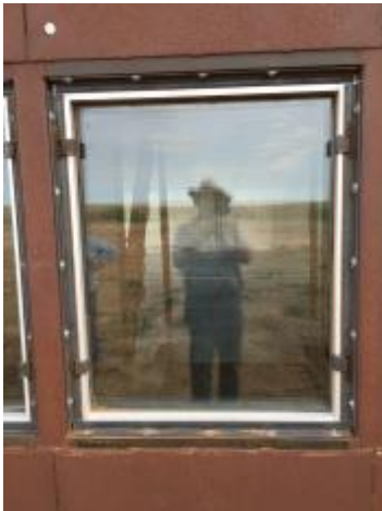
Figure C.9: Specimen 1-3 Pre-Blast Condition Exterior
