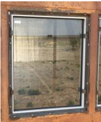
Figure C.41: Specimen 4-2 Pre-Blast Condition Exterior
