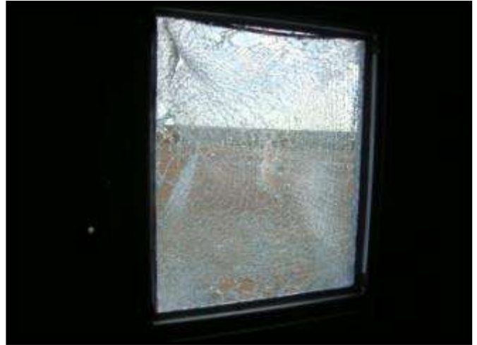
Figure C.18: Specimen 12 Internal Post-Blast Condition
