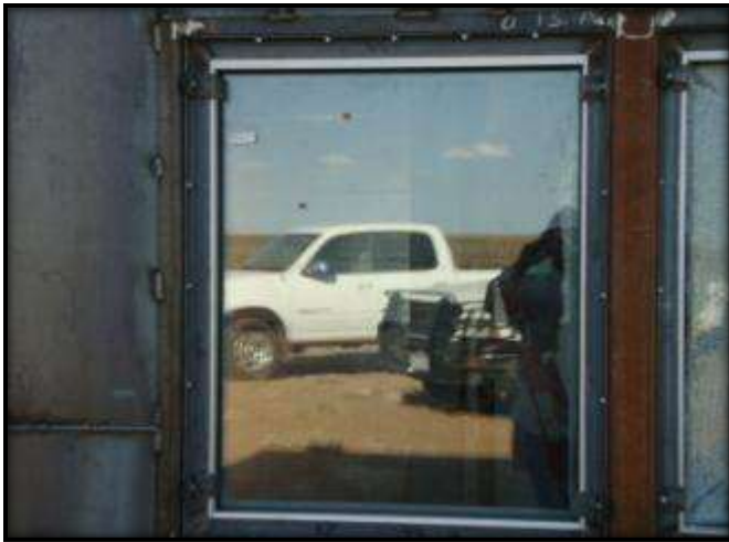
Figure C.23: Specimen 13 External Post-Blast Condition
