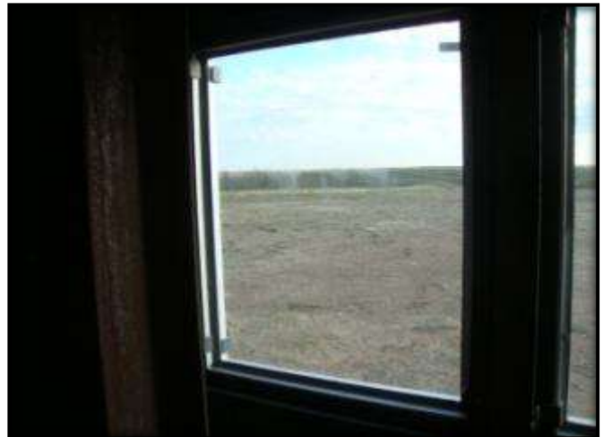
Figure C.30: Specimen 16 Internal Post-Blast Condition
