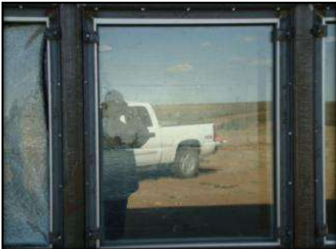
Figure C.25: Specimen 15 External Post-Blast Condition
