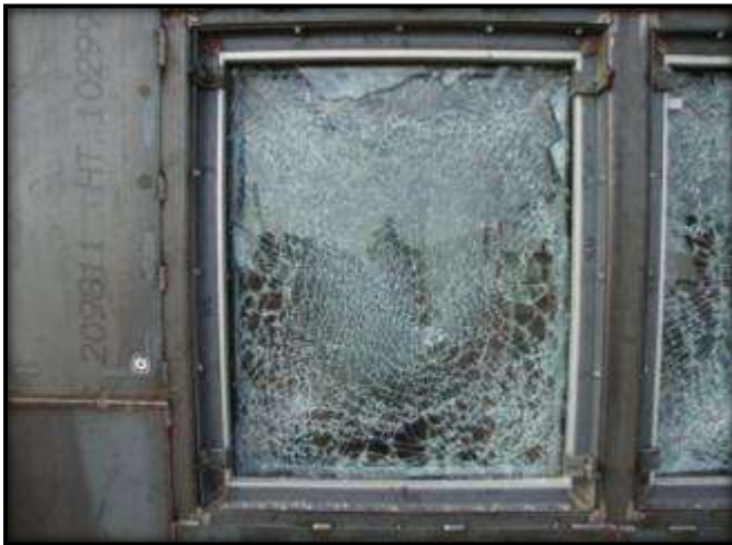
Figure C.11: Specimen 9 External Post-Blast Condition
