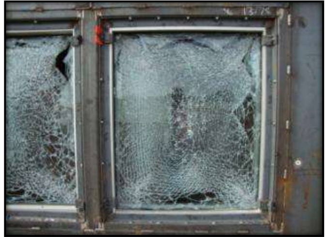
Figure C.14: Specimen 12 External Post-Blast Condition
