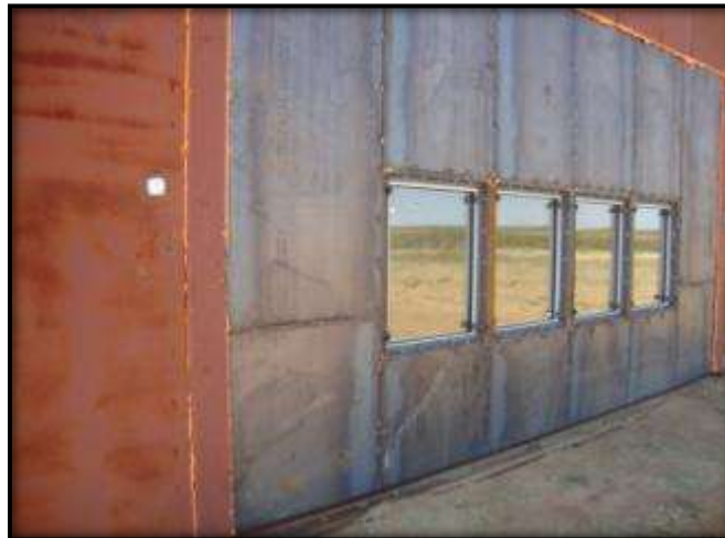
Figure C.19: Chamber 4 Pre-Blast Condition
